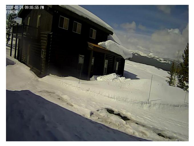
This is a photo of a small roof avalanche near Island Park. Warming temperatures cause water to percolate through the snow which lubricates the sliding surface. Roof avalanches have injured and killed people in the past, just one more thing to worry about. Photo: M.E.
